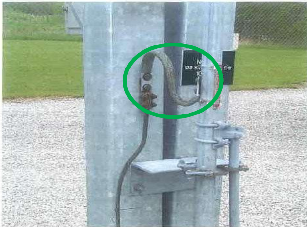
Figure 34—Typical braided ground
