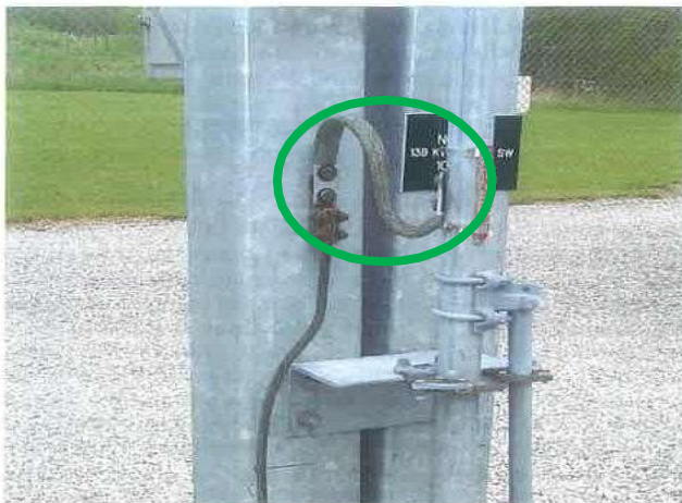
Figure 34—Typical braided ground
